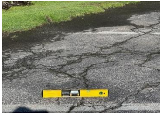
Southwest parking area, second space from the west, Running slope at front driver-side. Running slope at this location at 1%.
